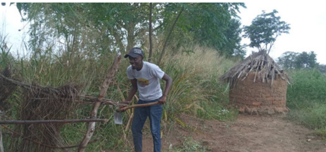
Tidying the compound of Gladys' ramshackle hut & repairing the urinal
